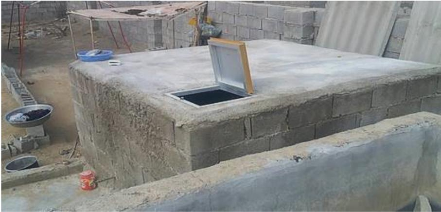
Fig. 4.4.9 Water container with concrete cover with hinged lid, Chabahar, 2013
