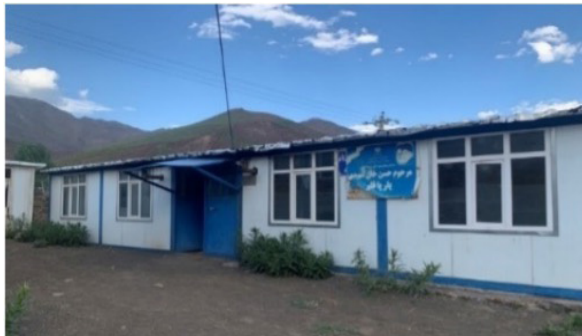
Photos: Samira Faridmanesh (Khoy, Jul 2023) Prefabricated classrooms
